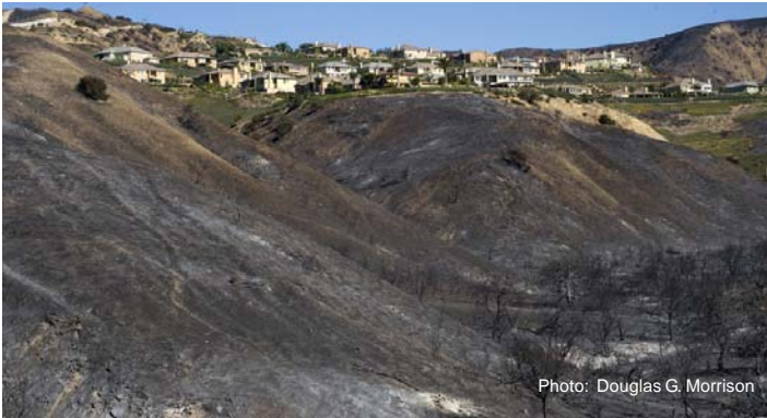
Brush clearance improves the chances that a structure will survive a wildfire.
